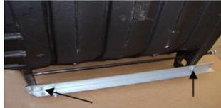
Attach 10mm bolts to the underside of the frame rails. These will be used to level the boiler. Screw the 4mm jacket affixing screw to the frame rail from the top down. Both the bolt and affixing screw will be located on the same end of the frame rail. The frame rail will then be bolted to the legs of the boiler with the frame rail end containing the affixing screw facing in the direction of the front end of the boiler.
