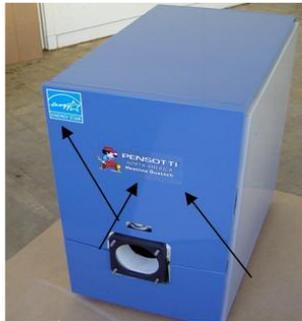
Upon completion of the jacket assembly the control unit can be mounted on the side of the boiler. The boiler is now ready for piping and connection to the fuel system, heating and domestic hot water, thermostat, and 110 Volt 60 cycle AC current.
